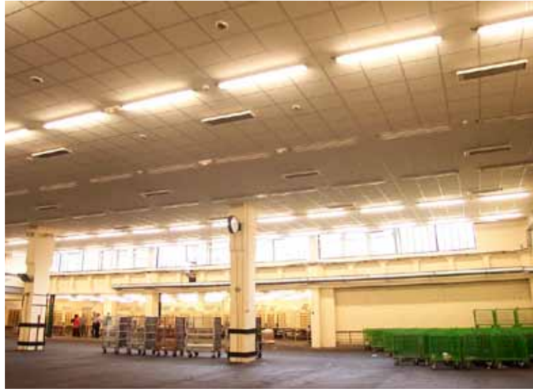
With radiant heaters, the heat is transferred to surfaces such as people, floors and fixtures. This creates comfort even in rooms with large volume.
