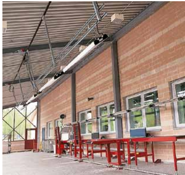
The IR heater can be mounted in an angled position to direct the heating where it is needed. Heaters used outdoors should be placed under a roof. In this installation the working stations are heated by IR heaters in the ceiling and CIR heaters on the wall.
