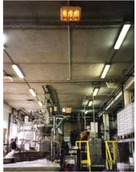
IRCFC is often installed in large warehouses. They give instant and effective heat which make them profitable quickly.
