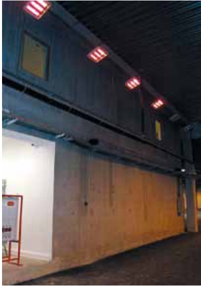
IRCFC can be mounted on the wall or on the ceiling and is suitable in buildings which are used sporadically like this go-cart track starting area.
