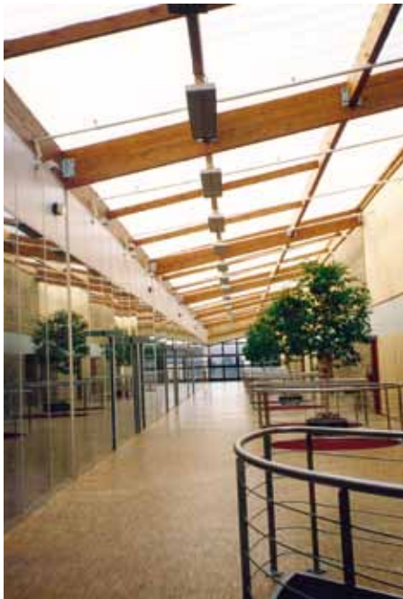
Corridors can be difficult to heat, but ceiling mounted EZ100 give off heat just where it is needed.
