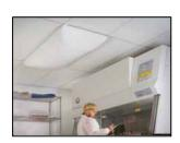
LabSox advantage is clear as air passes through specialized fabric panels resulting in uniform, low velocity, radially diverging air patterns with little if any turbulence.
