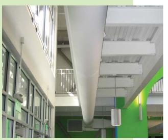
Traditional round fabric duct by DuctSox Corp.
